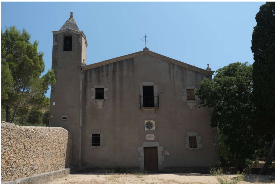
Figura 1. Façana principal (oest).
