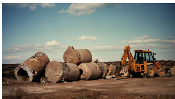
Photo 10. Left: 2002. North Malladeta beach and Brava beach. Removal of infrastructures. In the LIFE DUNA project, 270 man-holes with a depth ranging from 2.45 to 4.25 m were removed.
