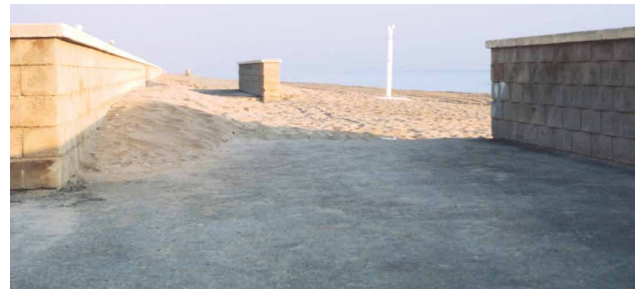
Photo 7. Detail of the sea promenade that stretched for 5.5 km to the south of the raised sea promenade and along the entire beach of La Devesa. It was formed by a 1.2-m high wall, which on the inside was joined to a road of some 5 m wide with accesses to the beach at specific intervals.
