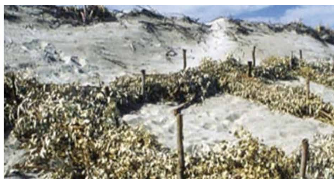
Photos 8 and 9. Trials with different types of material and arrangements to stabilise the sand. Left: Plastic meshes. Right: Bundles of eucalyptus branches originating from the removal of these trees.
