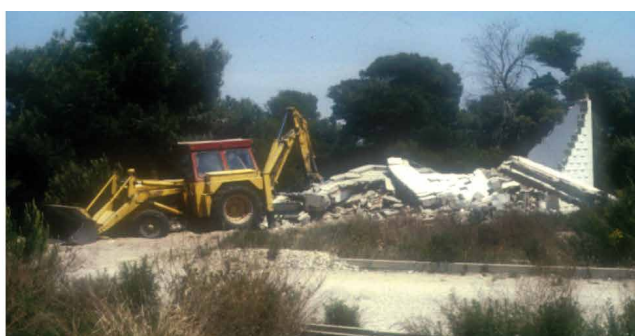
Photo 10. Left: 2002. North Malladeta beach and Brava beach. Removal of infrastructures. In the LIFE DUNA project, 270 man-holes with a depth ranging from 2.45 to 4.25 m were removed.
